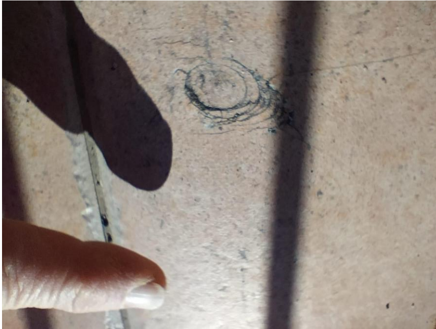
This tile on the balcony was damaged by impact of the meteorite. Credits: PRISMA/INAF
